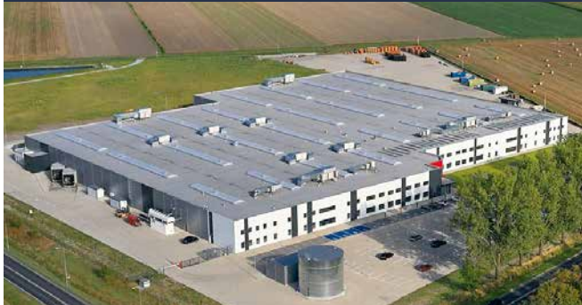
New fibre optic cable factory and new factory for specialized connectivity systems Rawicz, Poland
