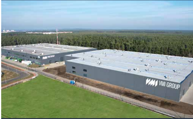
Expansion Tire Building systems factory Leszno, Poland
