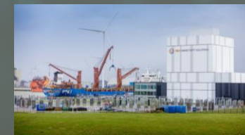
Eemshaven – new inter-array cable production facility
