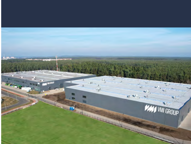
Expansion Tire Building systems factory Leszno, Poland
