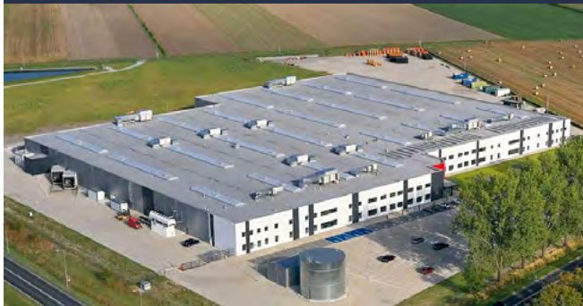
New fibre optic cable factory and new factory for specialized connectivity systems Rawicz, Poland
